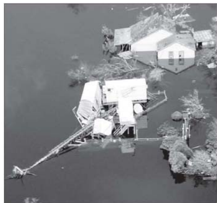
CELL tower falls on submerged home.
